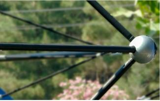
Metal parts are comprised of ST 37 Steel with a 3-step metal finish. Sandblasting and solvent-free zinc primer coating and electrostatic powder paint application is inherently corrosion resistant under extreme weather conditions and UV.
