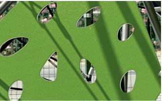
High quality panels made of HDPE panels are milled to provide a smooth, gently rounded edge. The thickness of the panels varies according to its purpose for floors, roofs, and walls.
