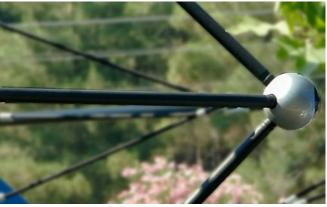
Metal pipes and other metal parts are comprised of ST 37 Steel with Metal finish; Sandblasting and treated with solvent-free zinc primer coating which is inherently corrosion resisted under extreme weather conditions and UV.
