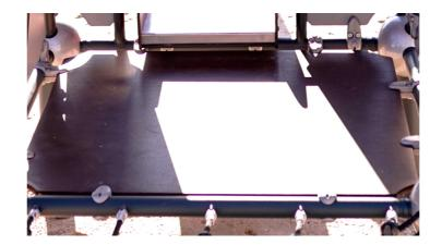
Durable and weatherproof laminated Plywood is used at platforms. These platforms have ability of anti-slip feature to increase the safety of the users.
