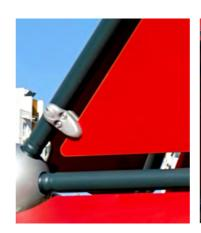
High quality panels made of HPL panels are milled to provide a smooth, gently rounded edge. The thickness of the panels varies according to its purpose for floors, roofs, and walls. These panels are connected to steel pipes or profiles with cast aluminum panel clamps or flanges. To increase the visibility of interior of the equipment, some panels are equipped with 5 mm thick anti-climb steel mashes. This wire mash is placed within either steel or HPL frame.
