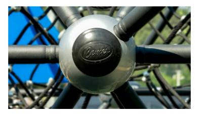
Single-casing aluminum cast spheres with anticorrosion treatment are placed at junctions. These spheres are designed with integrated bedding for connecting pipes.
