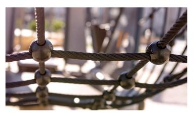
Single-casing, injection manufactured connectors are used at the intersection points of ropes.
