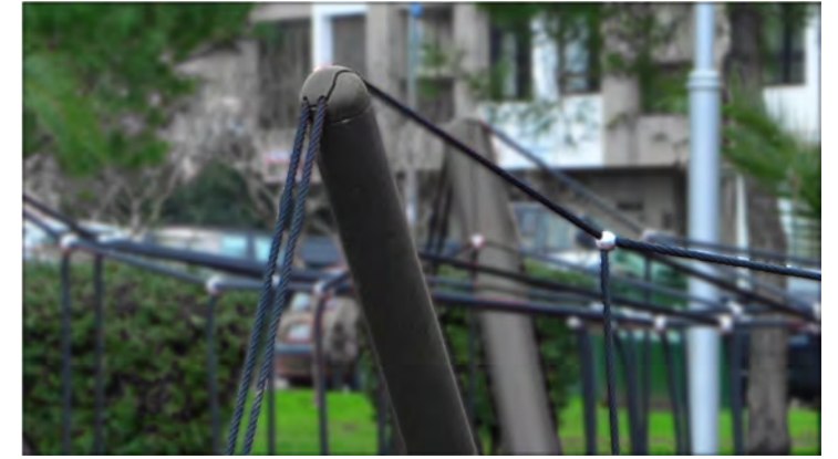
Single-casing aluminum cast caps have bedding channels in the cover system to keep the rope tight and stable.
