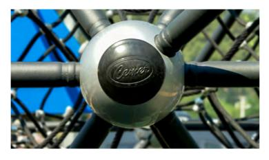
Single-casing aluminum cast spheres with anticorrosion treatment are placed at junctions. These spheres are designed with integrated begging for connecting pipes.
